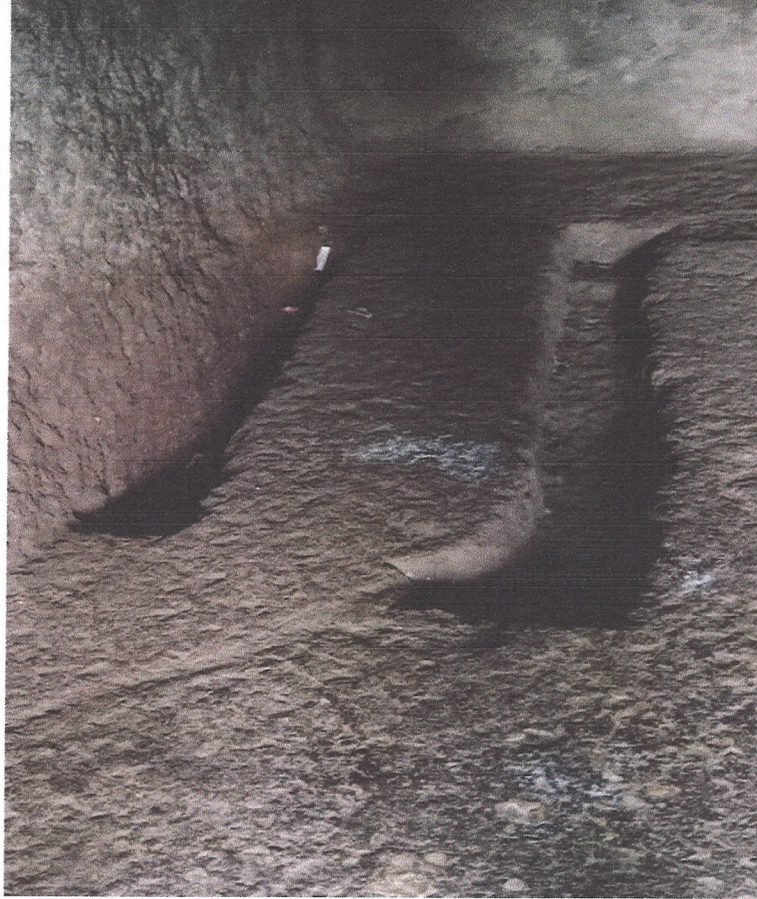
Measures taken for drainage of water in the class 'C' historical caves at vashala
